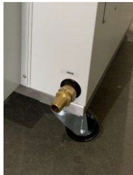
Fig 4. Location of 3/4 inch barbed drain.
