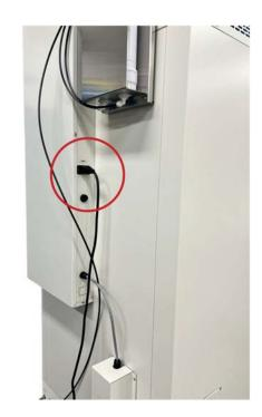
Fig 3. 15A/230V IEC socket location.
