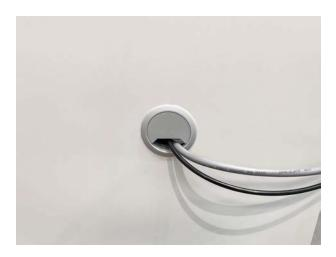
Fig 1. Power lead and water feed line passed through the lowest 54mm port hole
