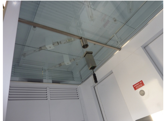
Above: Adjustable height Gro-Sensor with interior lighting
